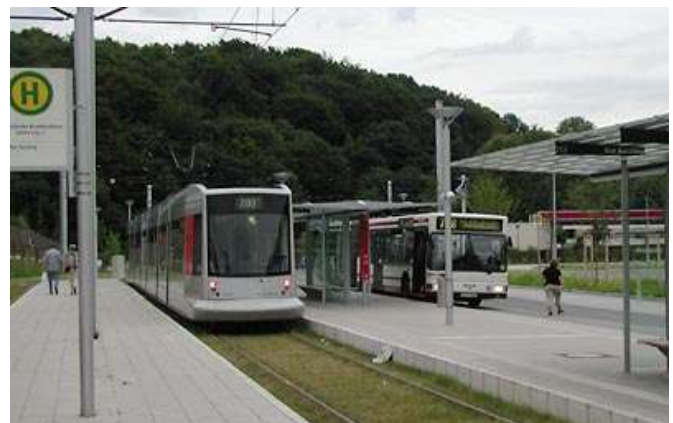
Light Rail and buses share the same platform. This is cost effective, but also offers the best passenger service where the change between rail and bus is necessary. Düsseldorf, July 2003.
